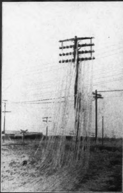
The severe ice storm which struck Amarillo, Texas, late in November left hardly a span of telephone or power lines undamaged. Upper left, a typical joint construction pole showing the tangled mess of wires left by the storm. Upper right, trees throughout the city suffered untold damage. Center, lines in the Santa Fe railroad yards. Below, other typical scenes.
